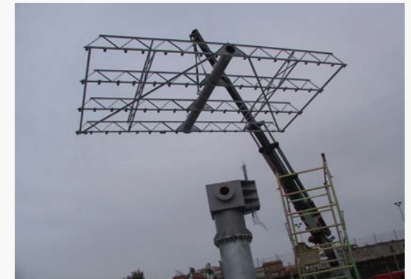
2: Installation of the right side of the supporting structure
