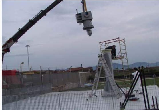
1: Reduction gears system box assembling
