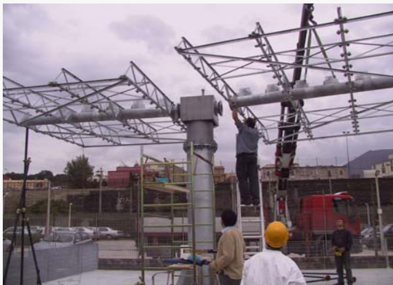
3: Installation of the left side of the supporting structure
