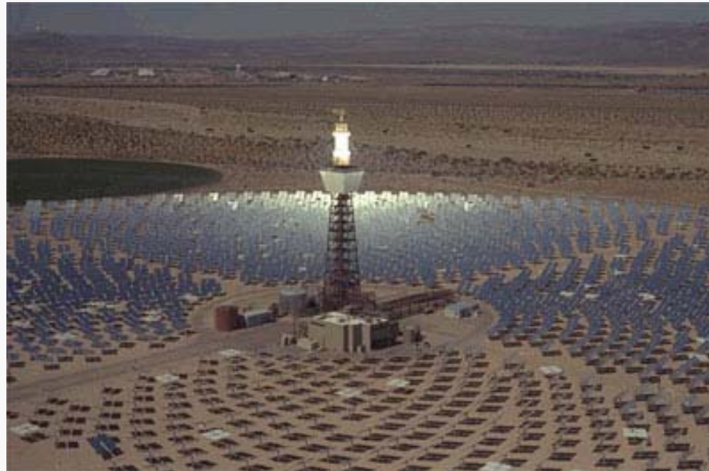
Solar Two Plant, 10 MWe (California, USA)
