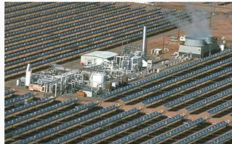
Linear parabolic collector plant at Kramer Junction (California)
