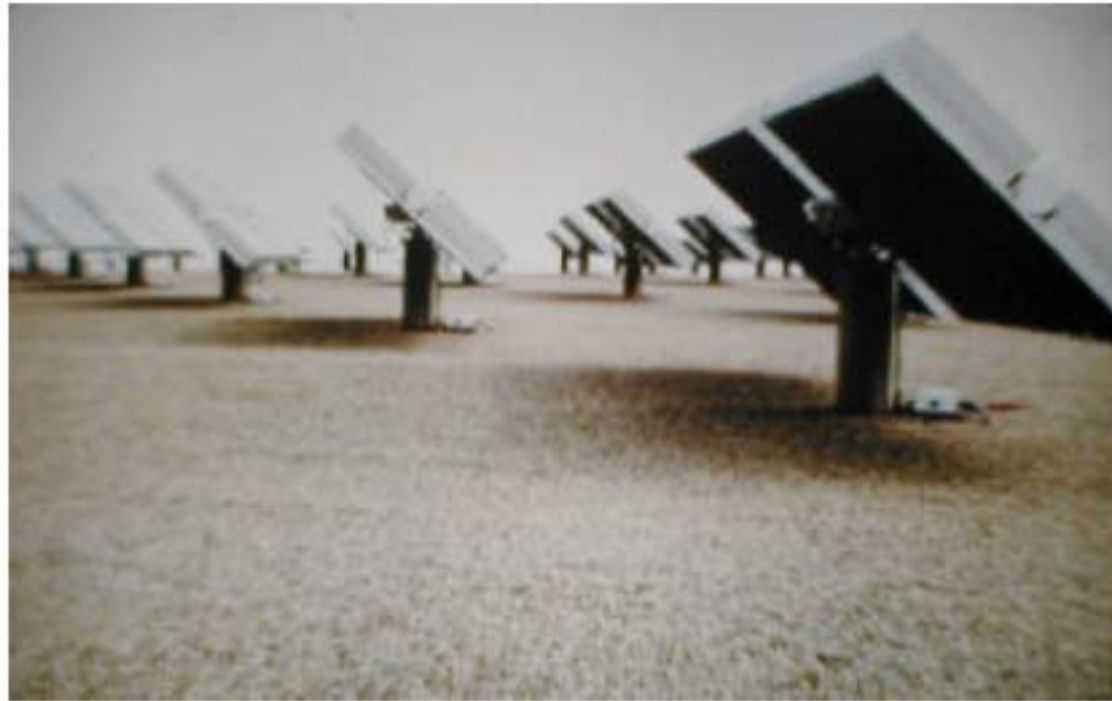
350 kW The modules include Point focus Fresnel lenses
