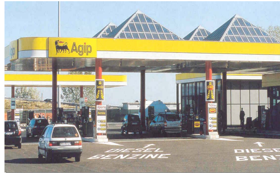
Italy, petrol station Grid connected
