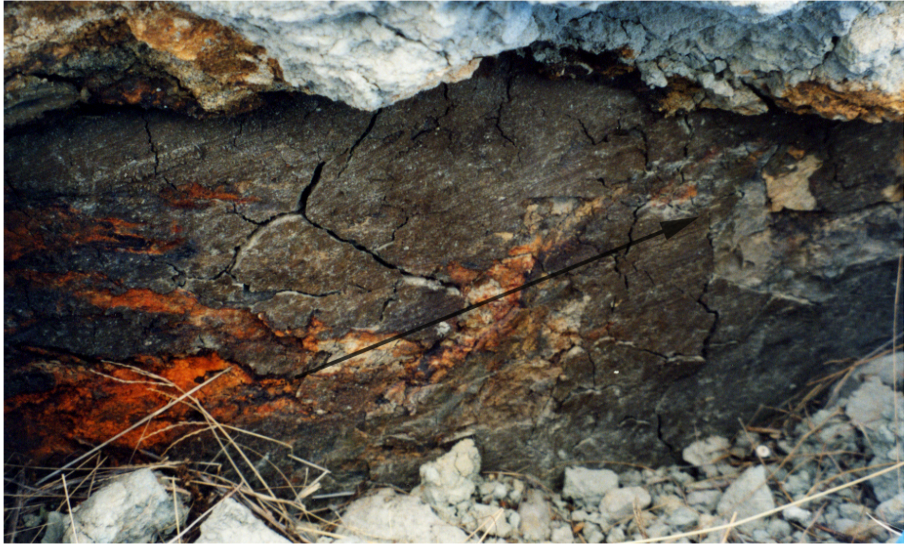
stripes on the fault plane
