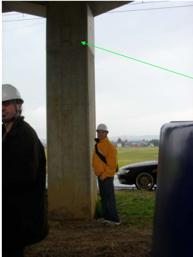
Mark of exploded mud water were found on bridge columns, where Sinkan-sen super express was derailed. Right: zoom
