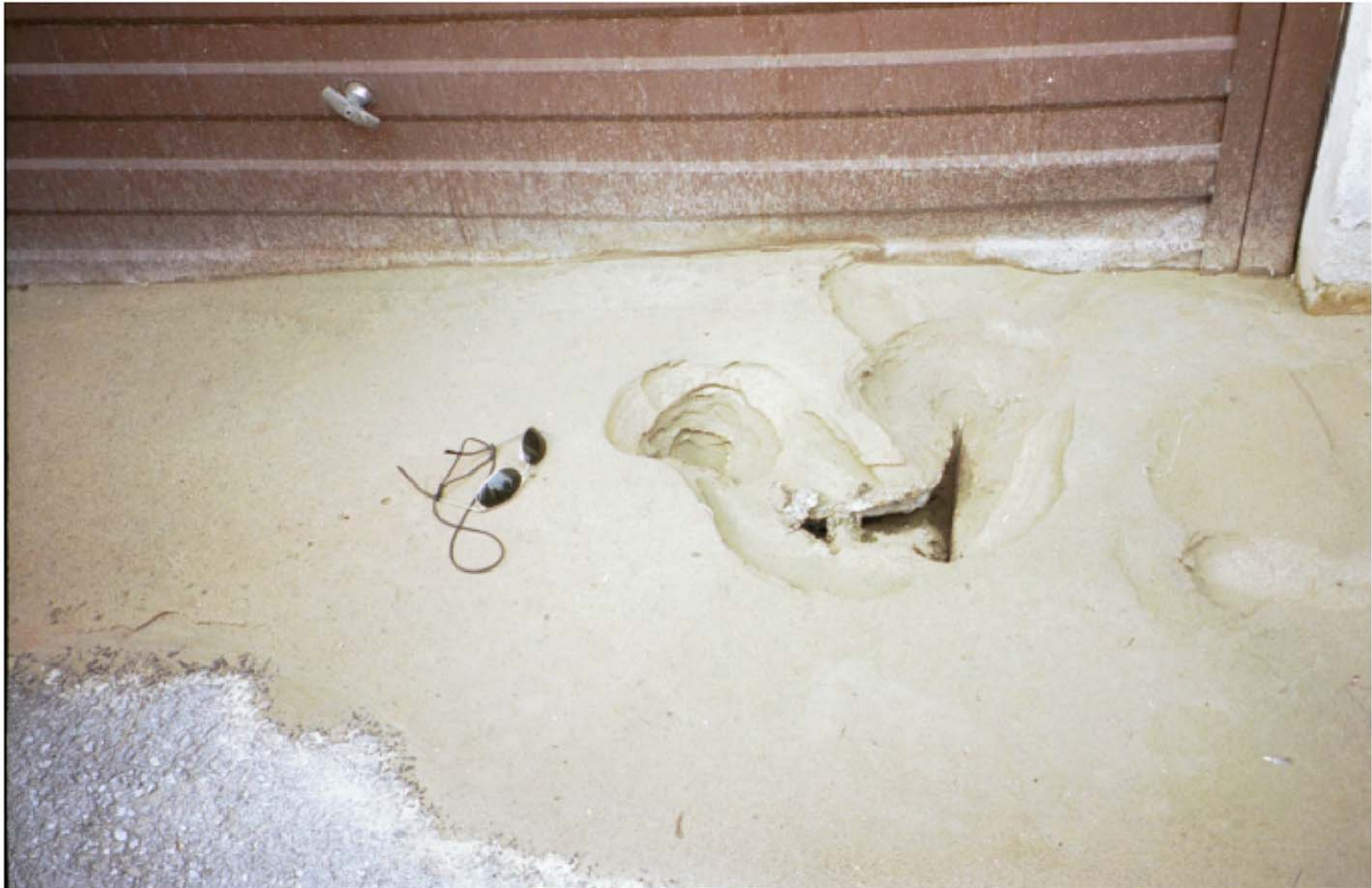
Sand boiling near the incline building
