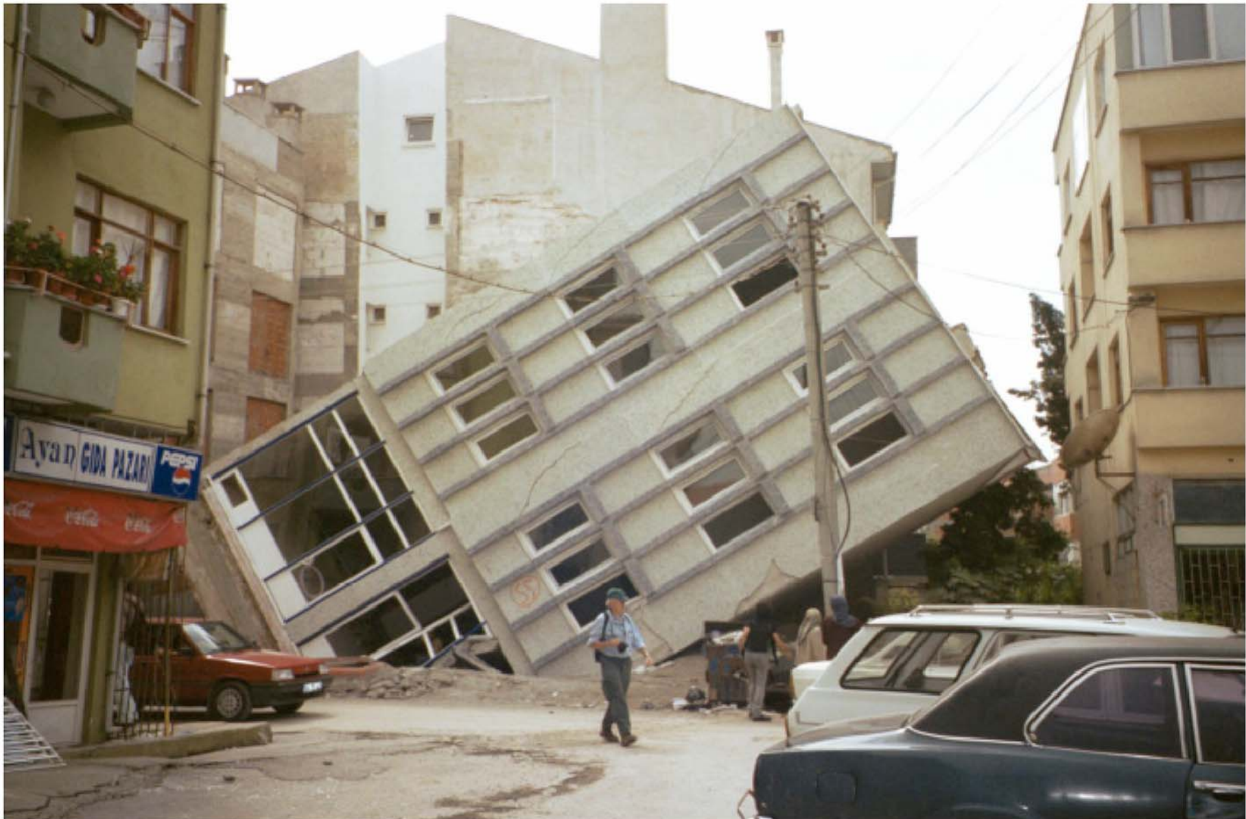
Incline building due to liquefaction during the Kocaeli earthquake
