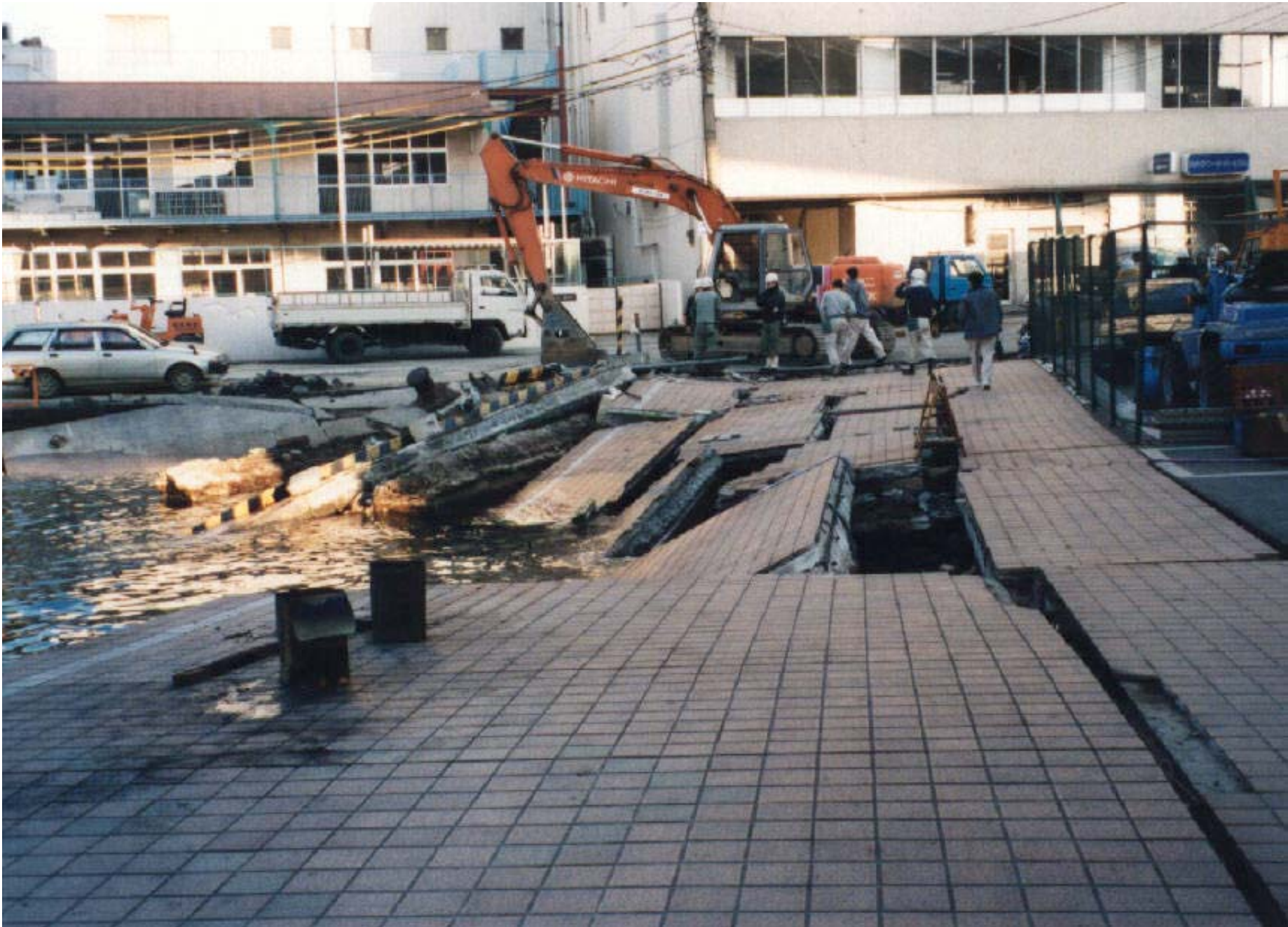
Damaged pier during the 1995 Hyogo-ken Nanbu earthquake
