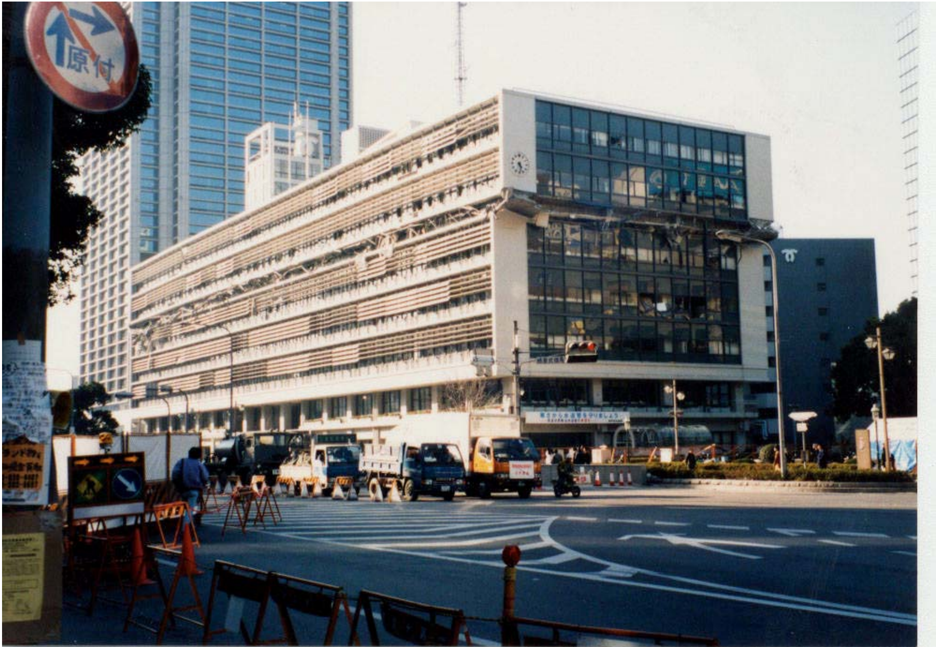
Damaged building in Kobe
