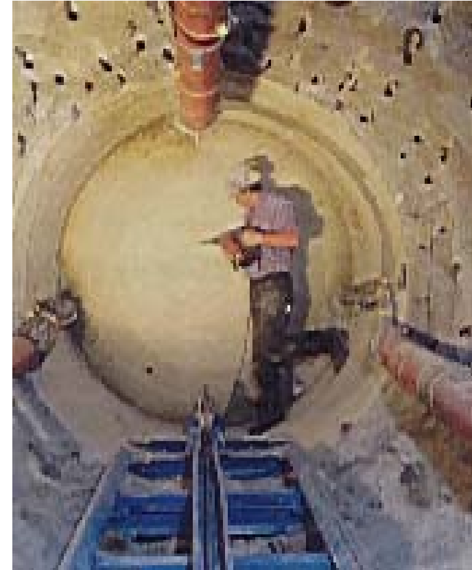
Emplacement of Clay Barriers Grimsel Test Site (GTS) Switzerland
