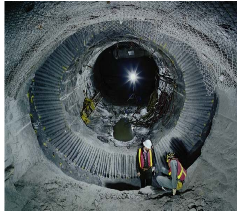
Construction of clay bulkhead for Excavation Damage zone (EDZ)
