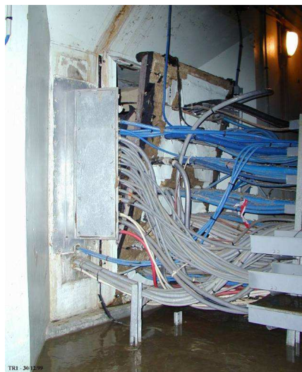
Figure 6 – damaged electrical penetration in the Unit 1 Fuel Building basement
