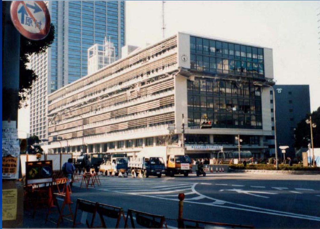
Damaged building in Kobe
