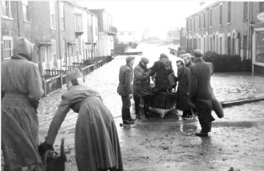
Storm surge in East Anglia UK, 1953
