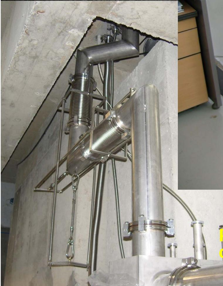
Pumping room (basement) vibration is isolated with double gymbal structures.
