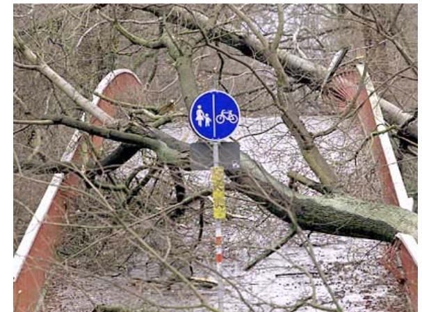
Storm damage by Lothar 1999
