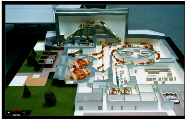
hadron therapy accelerator and gantry
