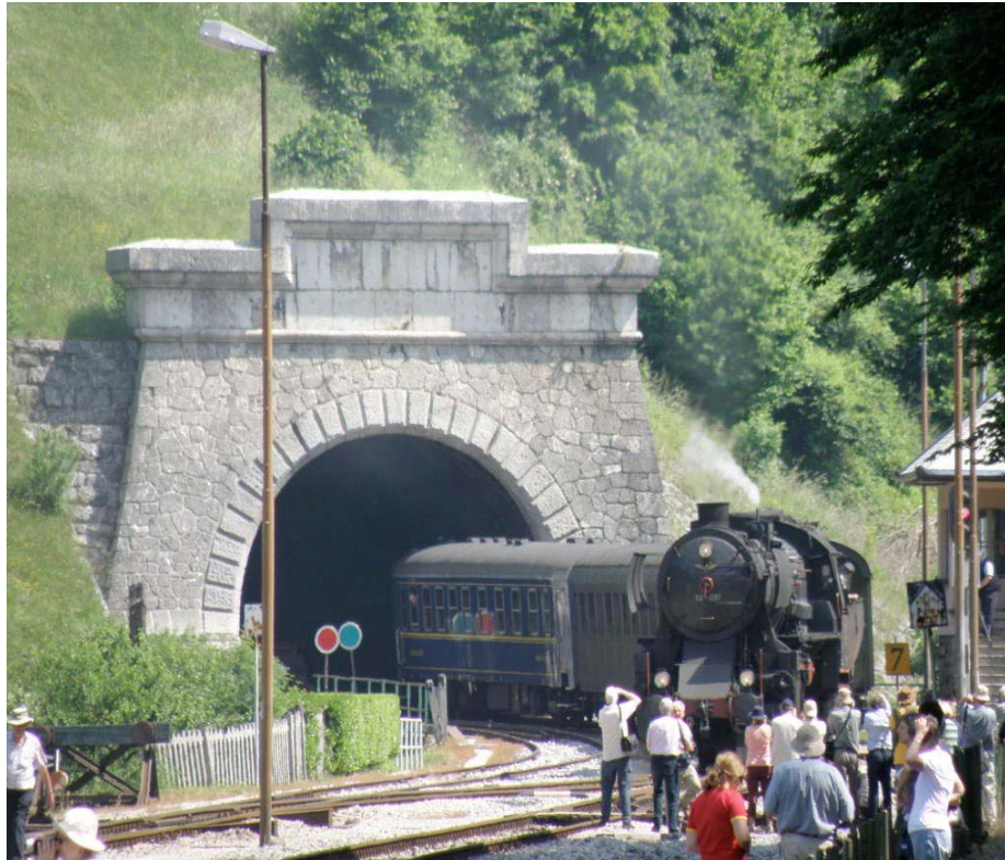
Bohinj railway tunnel at Podbrdo, Slovenia
