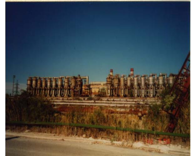
Evaporators at Aktau, Kazakhstan
