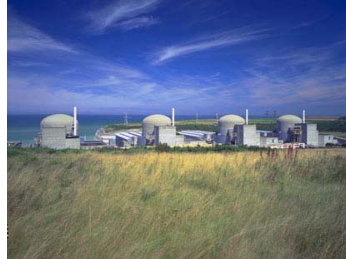
Paluel (F) nuclear power plant
