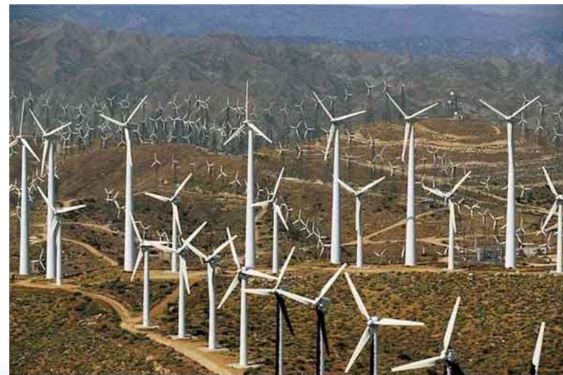
Palm Springs (US) wind farm
