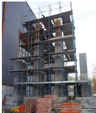
Construction of the large-scale bridge piers outside of the ELSA lab
