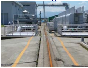
Crane rail near water discharge
