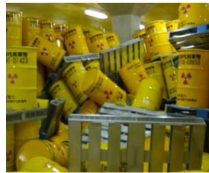
Inside of low level radioactive waste storage
