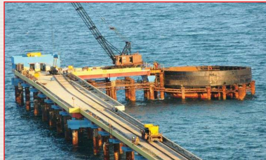
Lowering of Caisson in sea bed
