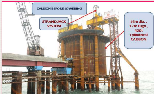
Lowering of Caisson in sea bed
