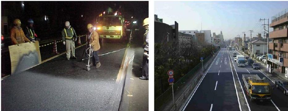
Fig. 6.7. Usage of TiO<sub>2</sub>-based photocatalytic material on roadway surfaces to convert nitrogen oxides (NO<sub>x</sub>) to nitrate: (left) application of the coating; and (right) finished roadway, with the coated surface showing a lighter color (courtesy of Fujita Road Construction Co., Ltd.).
