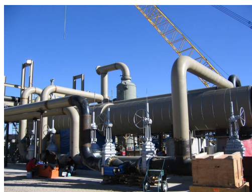
Geothermal fluid and evaporator
