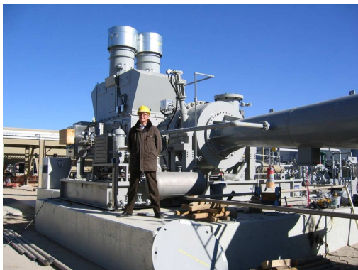
Expander and view of the geothermal field
