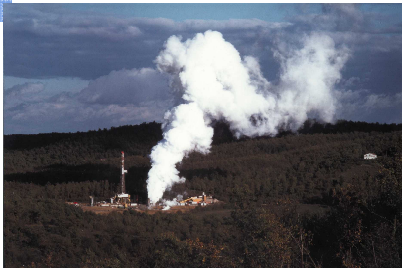
Montieri 1 well: 200t/h of dry steam → 20 MW, Italian Record
