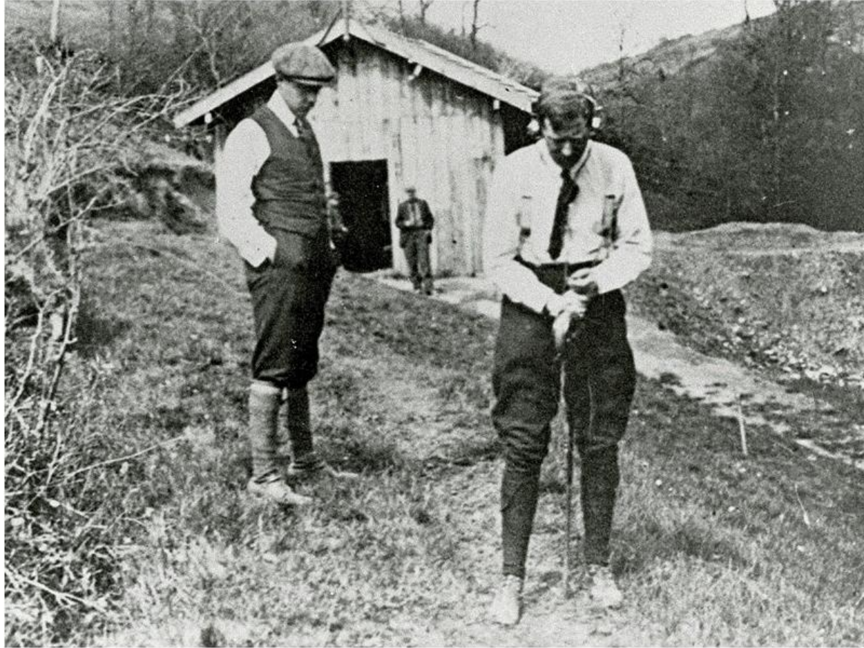
In 1912 Conrad Schlumberger, using very basic equipment, recorded the first map of equipotential curves in his Normandy estate near Caen.
