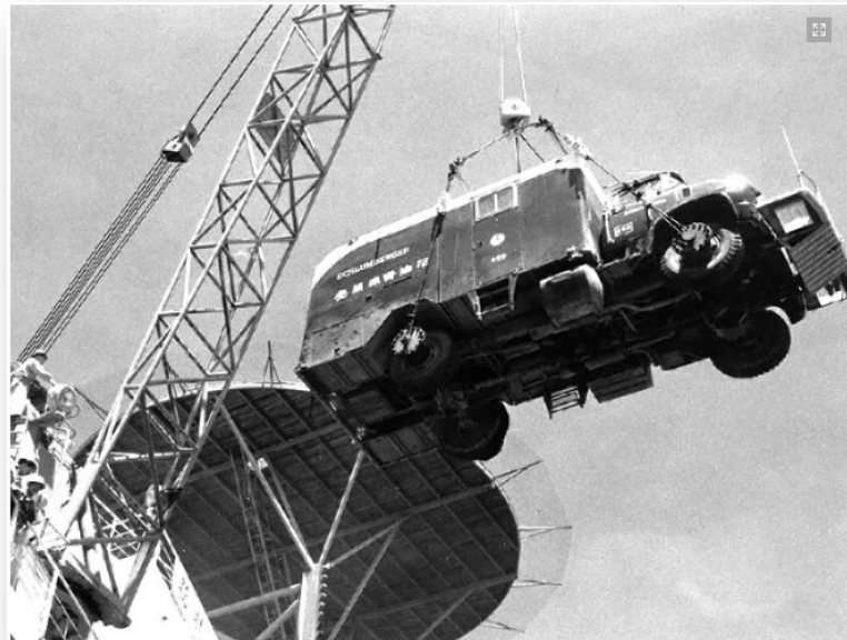
Logging truck being deployed for operations on an offshore drilling unit, South China Sea, 1947. The logging truck was substantially modernized, equipped with a winch and an electrical cable capable of operating a wide range of services in deeper and deeper boreholes.
