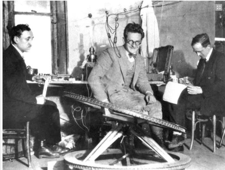
Marcel Schlumberger, far right, in the laboratory at Vitre, Brittany, testing a surface prospecting device used to measure dip.
