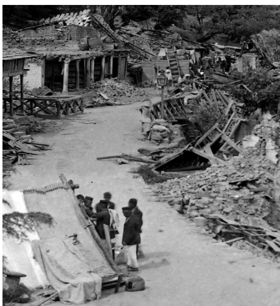
Dharmasala bazar in ruins following the 1905 M_w=7.8 Kangra earthquake. Photographed by Charles Middlemiss, Geological Survey of India.
