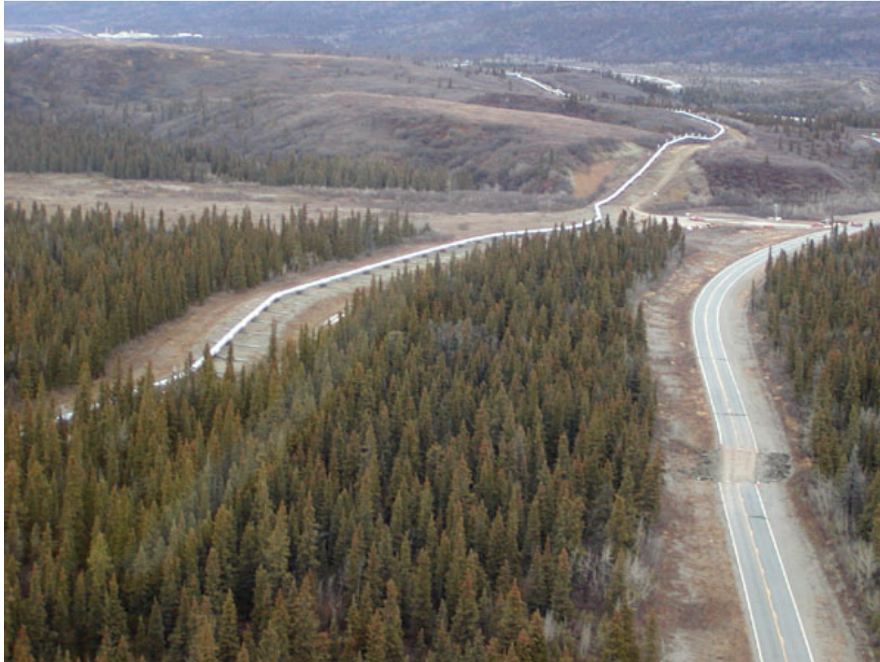
Trans Alaska Pipeline and Richardson Highway
