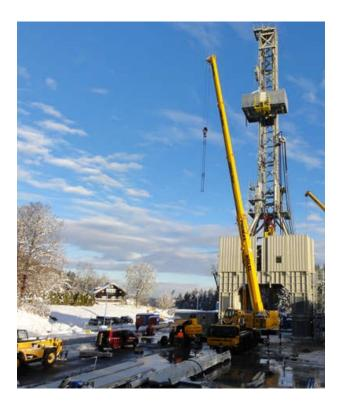
a EURO Benteq 450 rig was used (hookload capacity: 450 tons at 2,000 Brake-Horsepower) to drill the difficult, deviated well
