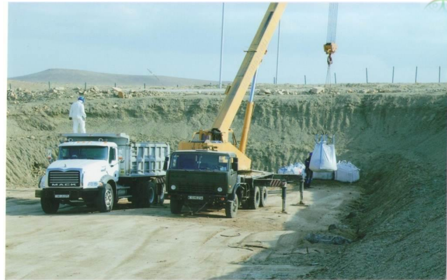
Loading contaminated soil to the trucks
