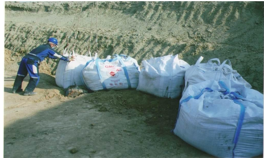
Loading soil to the sacks
