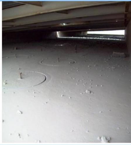
The monolith is a reinforced concrete structure of (36.2m long,10.5mwide and 6.1 m high) with 80 wells of 400 mm diameter and 4m height. The upper face of the monolith is 1.25 reinforced biological concrete slab (ric). Each well can take 7-8 st st bins for decay with a dose rate 2-1000 rem/hr. The plugs of the wells are 1.25( ric). Special drainage system for the wells is available.
