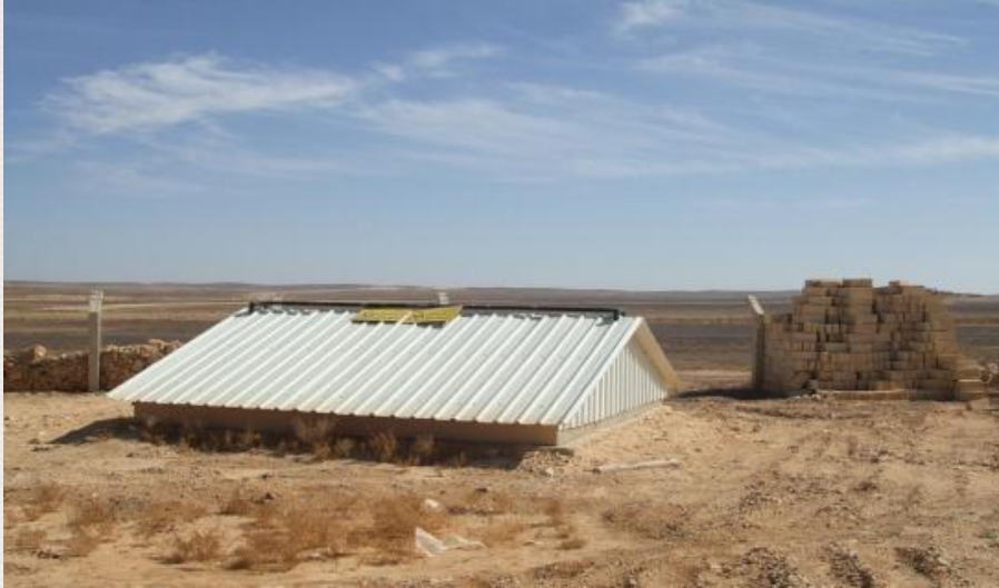
Reinforced concrete underground pit (3.6 m x3.6 m with depth 3.1 m) Capacity: 15 m 3
