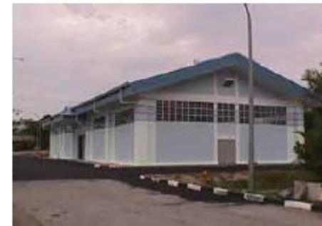
Storage 2 (Treated/Conditioned Waste)
