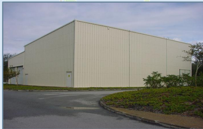
Building of Storage
